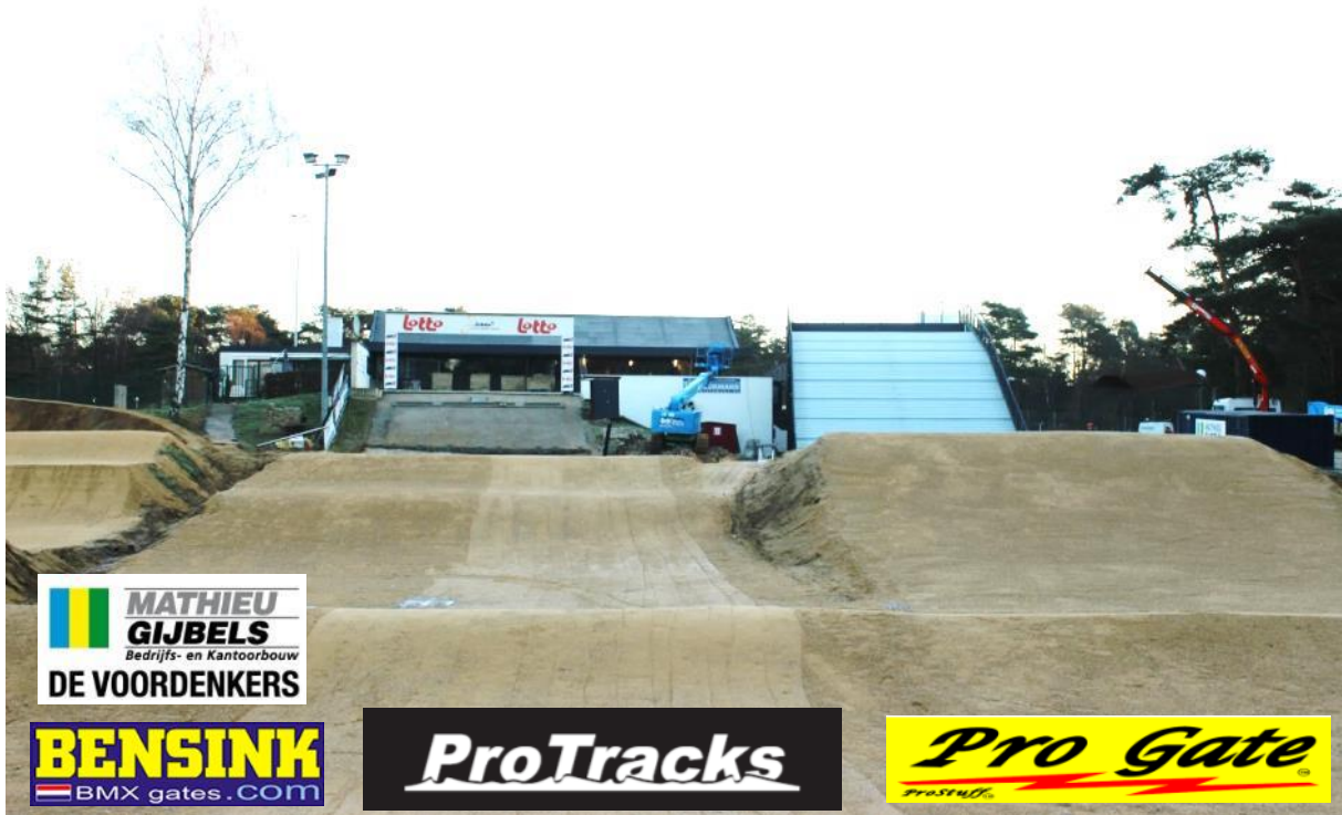
(track 5m/ 8m starting ramp Construction november 2013)
